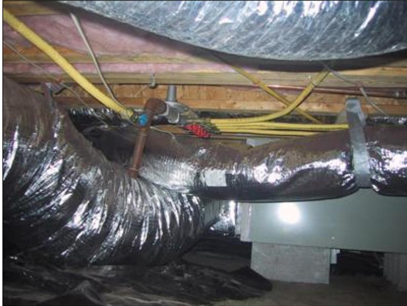
gas manifold in crawlspace underneath kitchen area and behind furnace
