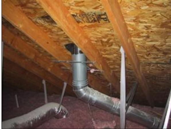
roof structure in attic (also showing vent pipe for water heater)
